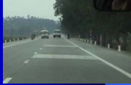
Rumble strips in Vietnam
